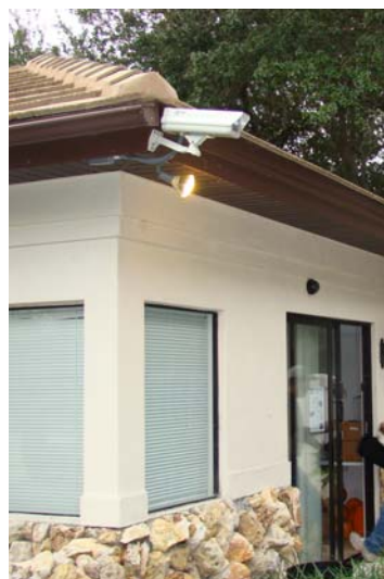
New security camera at Woodbriar gatehouse monitors pedestrian traffic in and out of Deer Creek.
